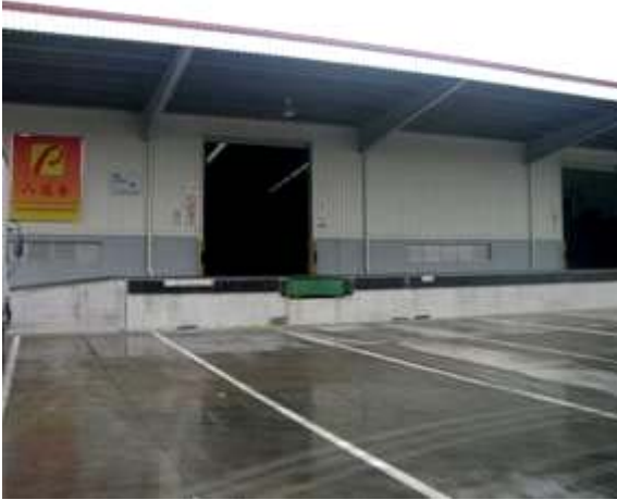
loading and unloading bay (80)
